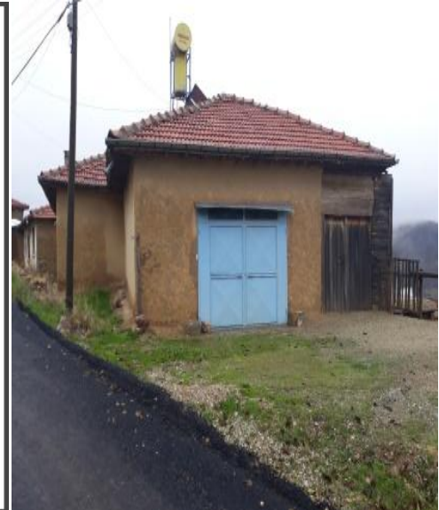
Figure 30. A roof with Marseille type tile in Seyituşağı
