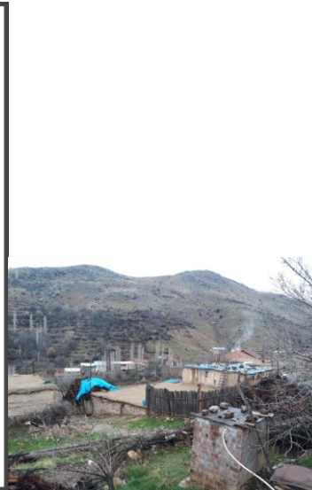
Figure 28. A flat roof in Seyituşağı
