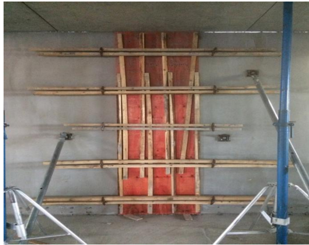
Fig. 7 Cast-in-site Connection between two Wall Panels
