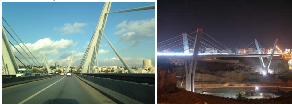
Figure 25. Modern Arab architecture (Abdoun Bridge).
