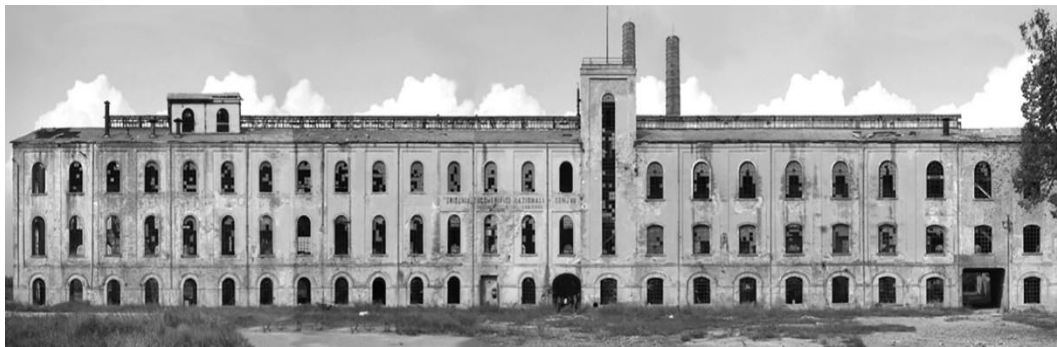
Figure 6. Codigoro sugar refinery. Principal building with serial repetition of the same element
