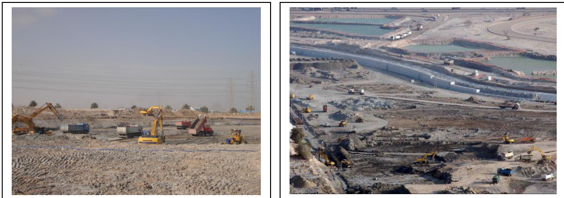
Figures(11&12)Site Photo - excavations activities
