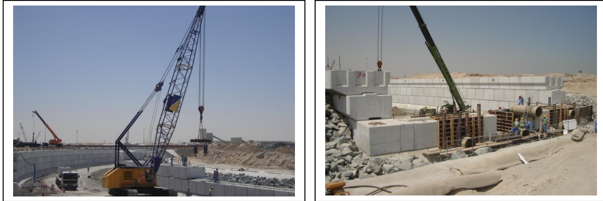
Figures (13&14)Site Photo Blocks placing
