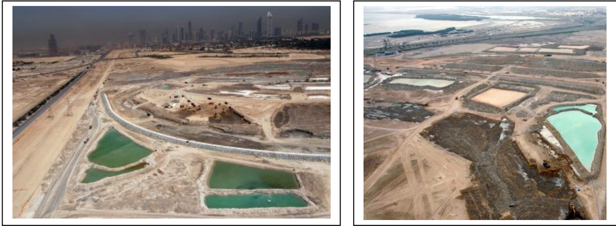
Figures9&10 Site Photo - dewatering ponds
