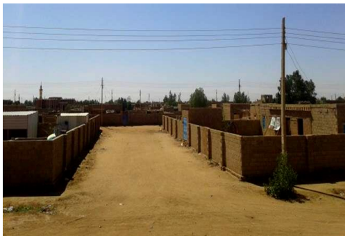
Photo 1: View of a cluster of low-cost houses
