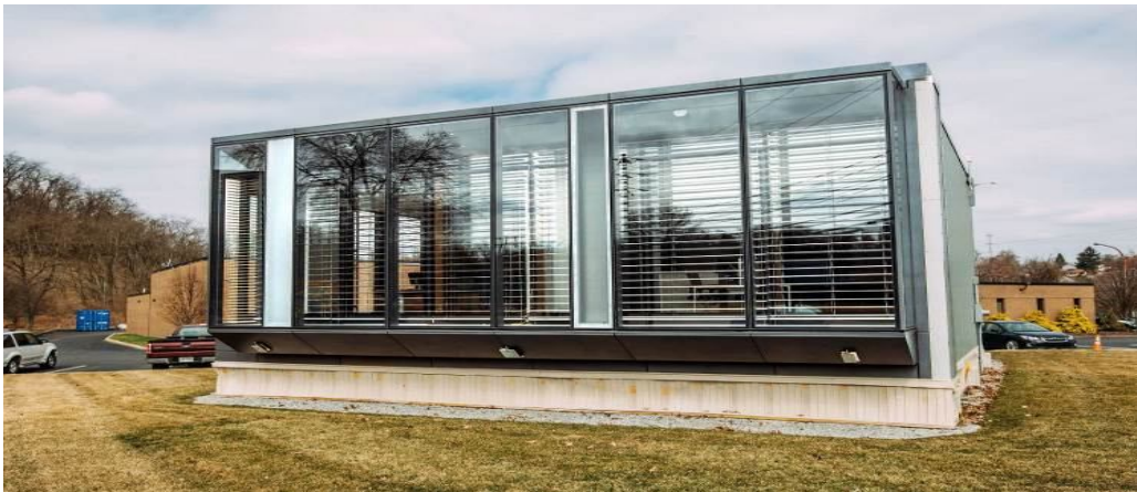
Fig. 10: Full-size Mockup testing daylighting louver system.
