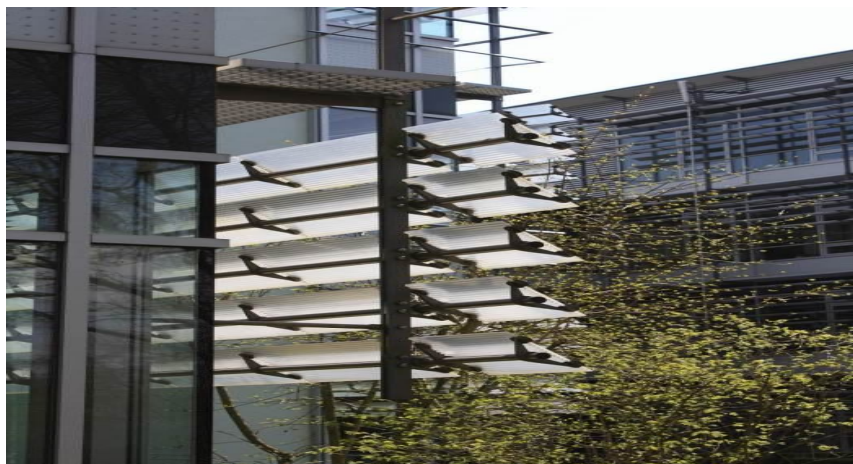
Fig. 14: Detail photo of the rotating prismatic panel's on the façade of the SparkasseFürstenfeldbruck office Building in Fürstenfeldbruck, Germany.
