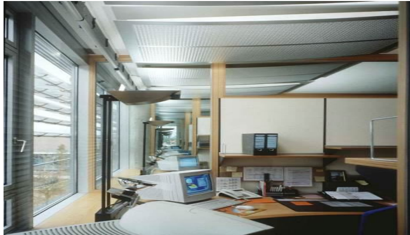
Fig. 15: Daylight deflection inside an office of the SparkasseFürstenfeldbruck Building, in Fürstenfeldbruck, Germany.
