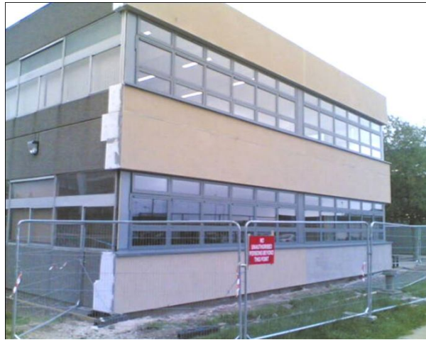
Figure 8: Retrofit of O Fiaich College, Dundalk 2008. (Photo: Coady Architects)
