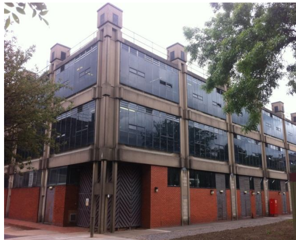
Figure 3: M&M Building, Birmingham University, by Phillip Dowson 1965 (Photo: O'Riain 2012)
