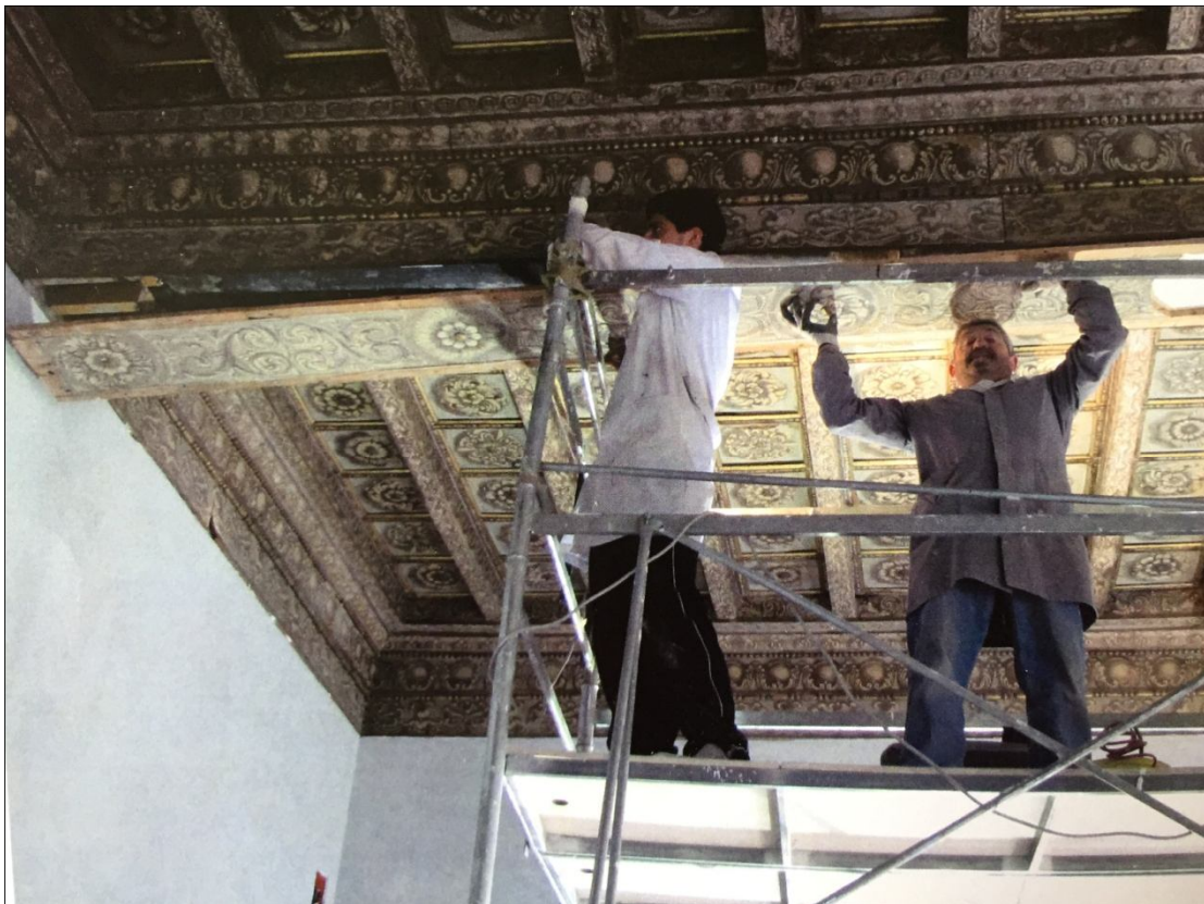
Fig. 2: Removing the Decorated Planks from the Main Wooden Beam
