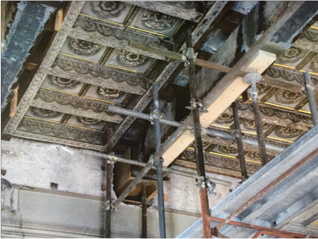
Fig. 4: Reinforcing the Beam Supports
