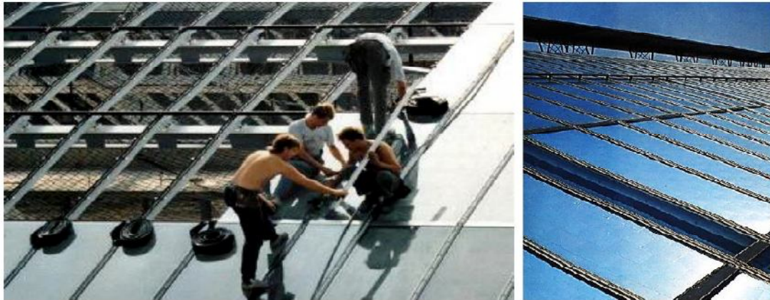
Figure 5: Exhibition Hall in Linz; Roof Panels
