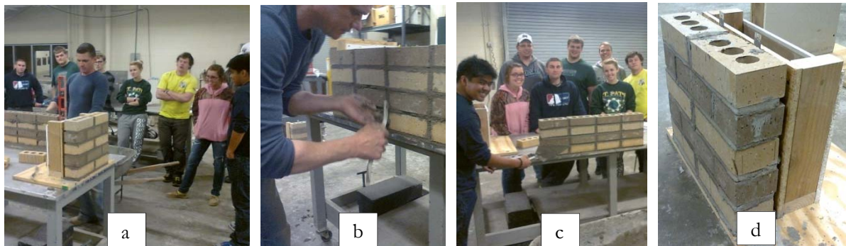
Figure 6: Mock-up Demo of Brick Veneer Over Timber Framing Wall in ArchE 2103 Course
