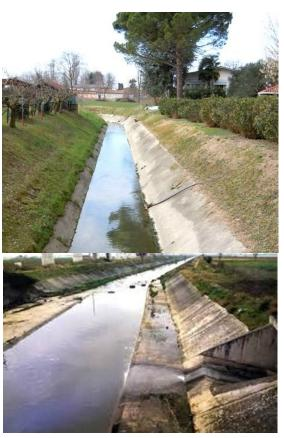
Fig. 10-11: Riverbed Concreting of a Stream and of the Regi Lagni near Caserta
