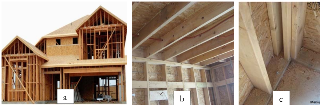
Figure 9. Timber Framing System (a) (Url 8, 2012), (b) and (c) Photograph by Semih G. Yildirim, Kumburgaz, Istanbul
