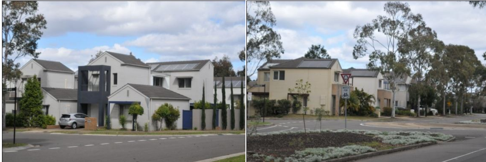
Figure 5: Solar Panels of Residential Houses in Newington
