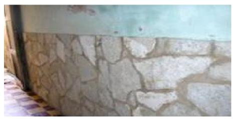
Figure 4: Flagstone Veneer Buildings in the Historic Center Santiago. Note the Capillary Phenomenon over the Slabs
