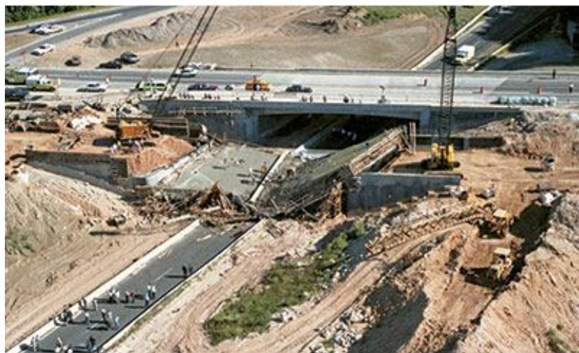
Figure 1: Collapse of Bridge No. 4 in 1989
