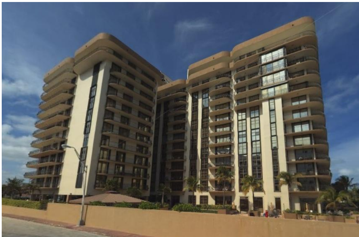
Figure 1. Champlain Towers prior to the collapse of the south tower. The portion of building that collapsed is on the right.
